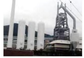
2 Heritage related to Yahata Steel Works
